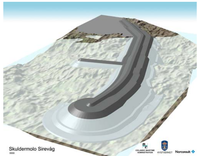
Figure 2. The Sirevåg berm breakwater
