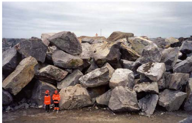
Figure 3. Sirevåg berm breakwater, stock pile of stone classes I and II
