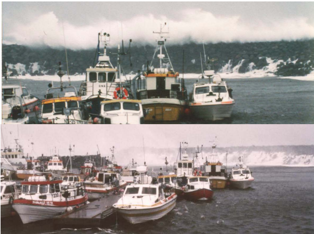
Figure 15. Rear side of the Bakkafjordur breakwater during a storm in 25 October 1995, overtopping over the crest and through the crest.
