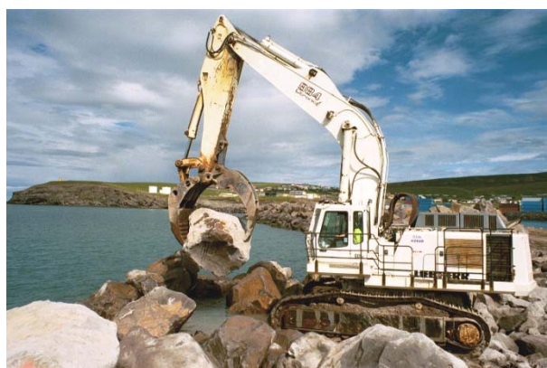
Figure 4. A 110 tonne excavator working on a level of Class IV rock of 1 to 4 t rock, placing Class I of 16-30 t at the head of the Husavik berm breakwater, Iceland.
