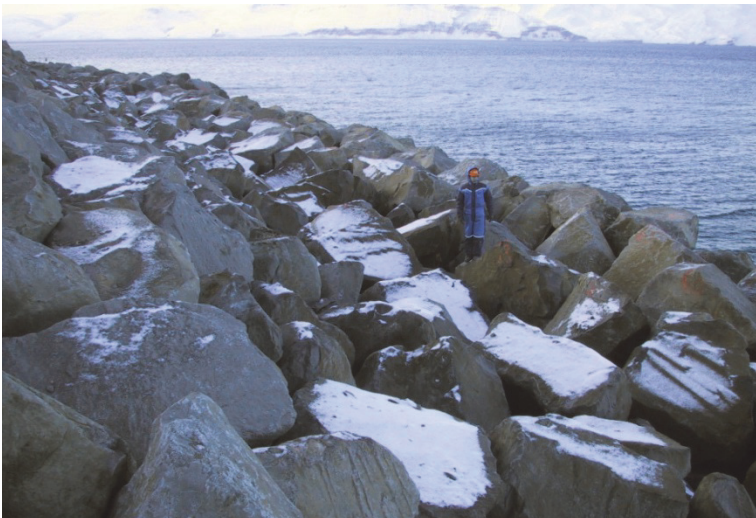
Figure 7.11. Narrowly graded stones on the Husavik berm breakwater, Iceland. Classes I and II, 16-30 t and 10-16 t.
