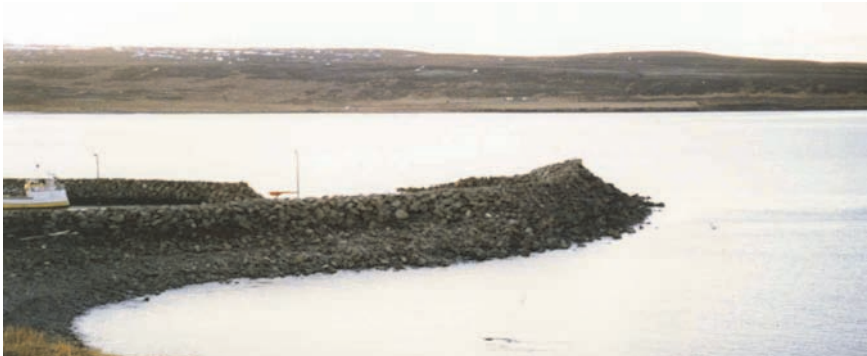
Figure 9.37. The Bakkafjordur breakwater reshaped after the storm of October 1995 into the crest, but did not breach.
