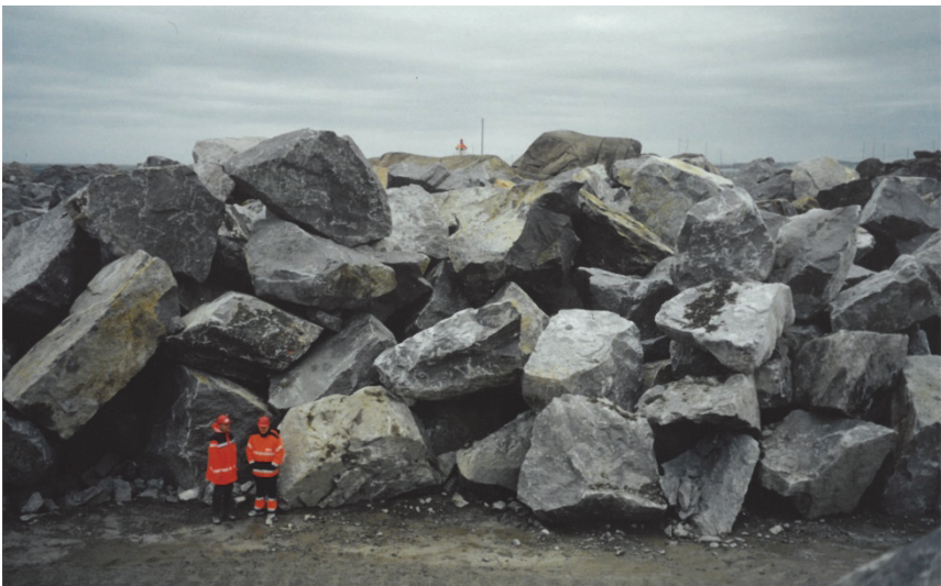
Figure 6.5. Stockpile of Class I, 20–30 t, and Class II, 10–20 t, armourstone for the Sirevåg breakwater.
