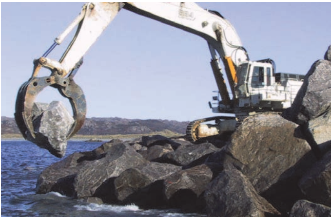
Figure 5.4. A 110 t excavator working on a level of Class IV rock of 1 to 4 t rock, placing Class II of 10–20 t at the submerged part of the roundhead of the Sirevåg berm breakwater, Norway.
