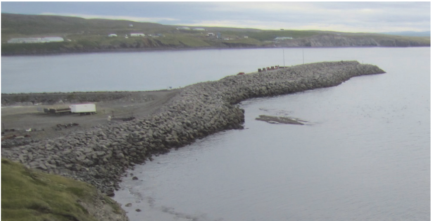
Figure 9.17. The partly reshaping Icelandic-type berm breakwater at Husavik 14 years after construction. Based on 3D physical model study, the shallows at the root of the breakwater cause wave breaking and high wave forces that were avoided with the breakwater alignment.
