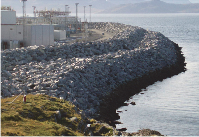
Figure 9.14. The Icelandic-type berm structure protecting the Hammerfest LNG plant, Norway. Photo taken in 2008.
