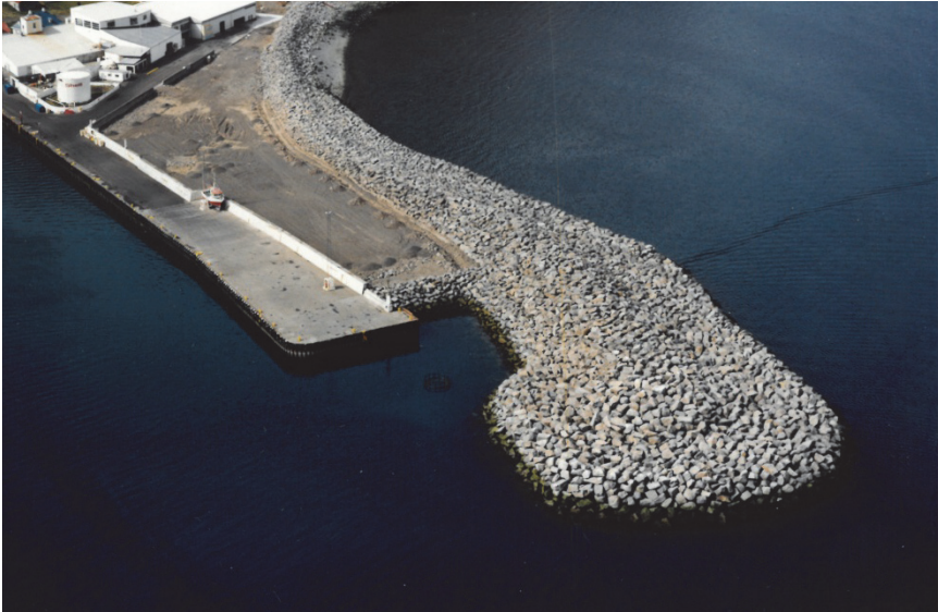
Figure 5.21. The Bolungarvik breakwater.
