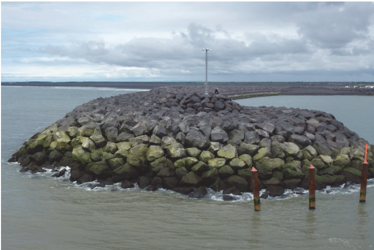
Figure 5.19. Example of an Icelandic-type berm breakwater at Landeyjahöfn with similar rock 12–30 t at trunk and head section.
