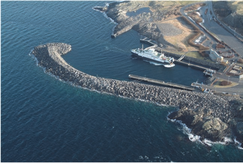
Figure 9.42. General view of the Mortavika Breakwater and harbour after the 2005 storm. The rock was quarried from the paved area in the upper right of this image. Notice that the breakwater trunk is extensively reshaped, while the breakwater head, which is not as exposed, has retained its shape. Courtesy of Norwegian Public Roads Administration.
