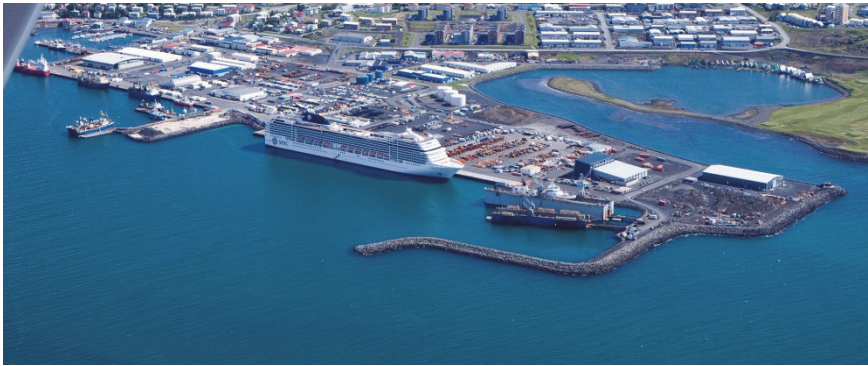
Figure 5.22. The breakwater in the Port of Hafnarfjörður shelters a multipurpose quay and a ship repair basin with floating docks. From the land area the breakwater starts with a northerly direction, then turning towards east, before the end is turned toward north-east. Photo by Mar Sveinbjörnsson.
