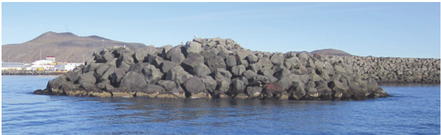
Figure 5.20. The roundheads of the two Grindavik berm breakwaters, partly reinforced at the harbour side with 13 to 28 t armourstone.
