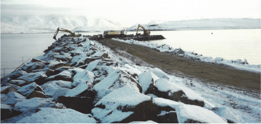
Figure 9.2. Construction of the Dalvik breakwater during the winter 1994 to 1995.
