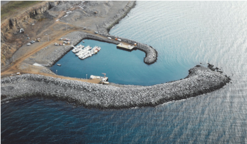
Figure 9.34. The Bakkafjordur harbour in the summer of 1995. A leeward breakwater was constructed in 1989.
