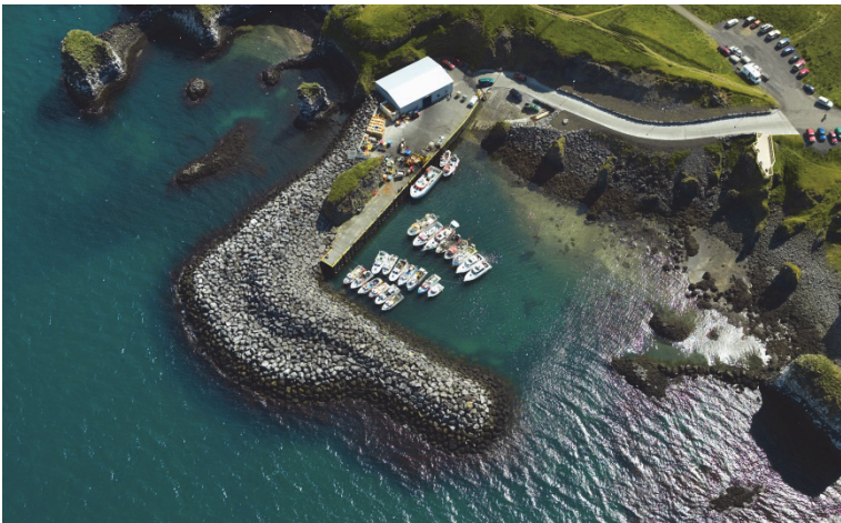
Figure 1.7. The berm breakwater at Arnarstapi, Iceland, sheltering a small fishing harbour. Photo by Mats Wibe Lund.
