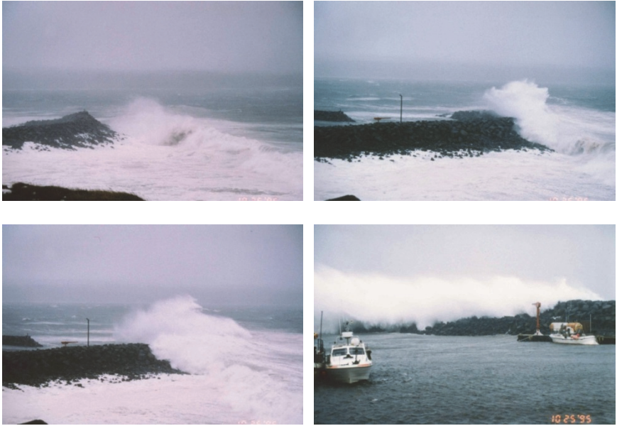
Figure 9.35. Waves breaking in front of and over the Bakkafjordur breakwater during the storm of October 1995.
