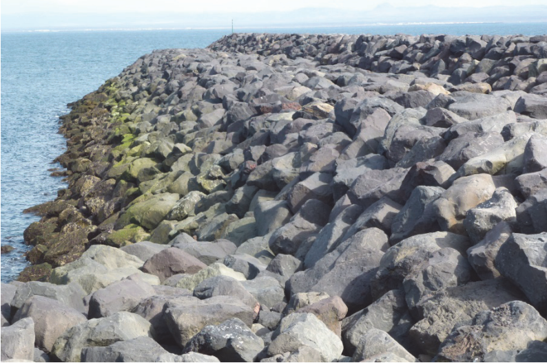
Figure 7.9. Extension of Helguvik with special placing of Class I rock.
