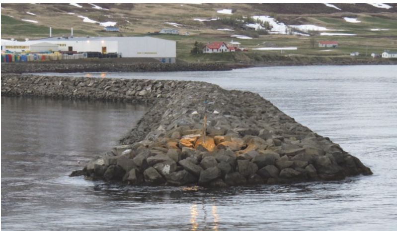
Figure 9.4. The Dalvik breakwater. Photo by Haraldur Gudjonson.
