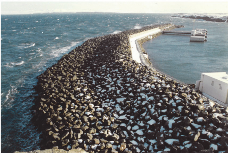
Figure 1.2. Berm breakwater of Helguvik, Iceland. Designed in 1983 by Baird & Associates and constructed in 1986-1988 by Icelandic contractors.
