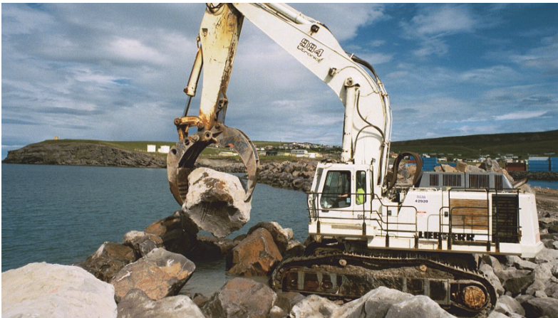
Figure 9.16. Excavator placing Class I 16–30 t stones on the head of the Husavik berm breakwater, Iceland.
