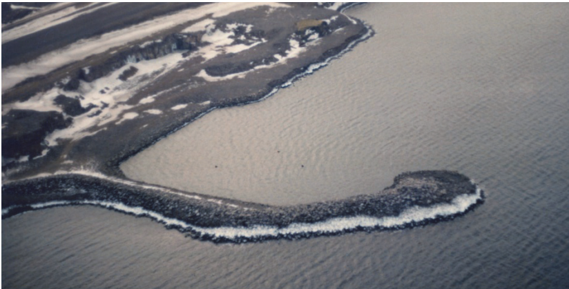
Figure 9.28. The Bakkafjordur breakwater and the local quarry in February 1986.
