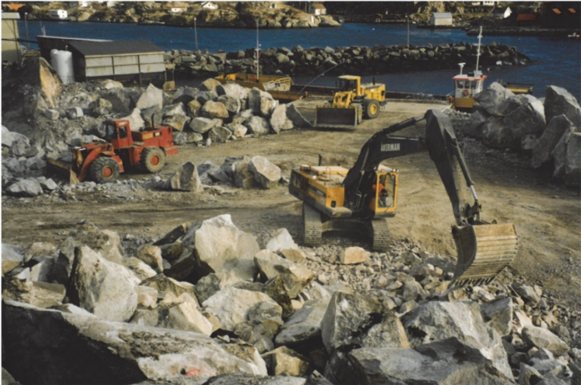
Figure 7.3. Loading a split barge with quarry run by wheel loaders. Sirevåg breakwater.
