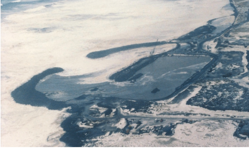
Figure 9.23. Aerial view of the St. George breakwaters when near completion during a severe storm evaluated as equivalent of the design storm at the time. Photo and information by J. Gilman.
