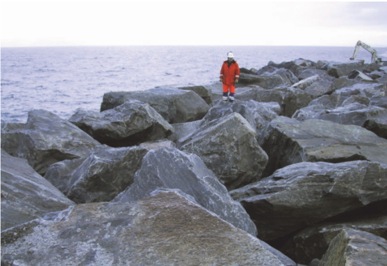
Figure 7.13. Class I stones, 20–35 t on top of the Icelandic-type berm of the breakwater protecting the Hammerfest LNG plant, Norway.
