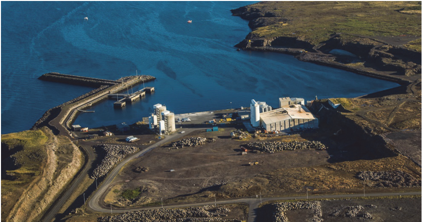
Figure 9.6. The new hardly reshaping Icelandic-type berm breakwater at Helguvik, connected to the old partly reshaping mass-armoured berm breakwater. Photo by Haraldur Gudjonson.
