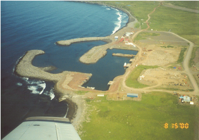
Figure 9.22. The St. George berm breakwaters; an aerial photo from the year 2000. Photo by J. Gilman.
