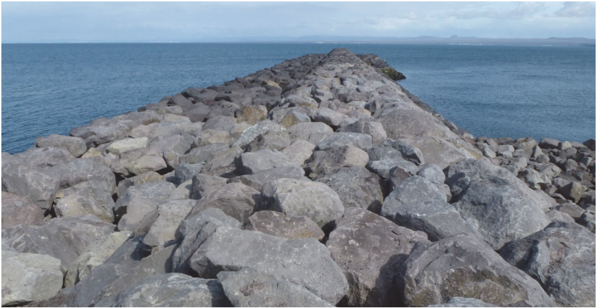
Figure 9.7. The new hardly reshaping Icelandic-type berm breakwater at Helgukvik.
