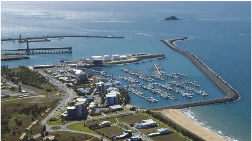
Figure 9.47. Mackay harbour, the Small Craft Harbour breakwater to the right on the photo protecting the marina that was built adjacent to the South breakwater. Photo by North Queensland Bulk Ports Corporation.
