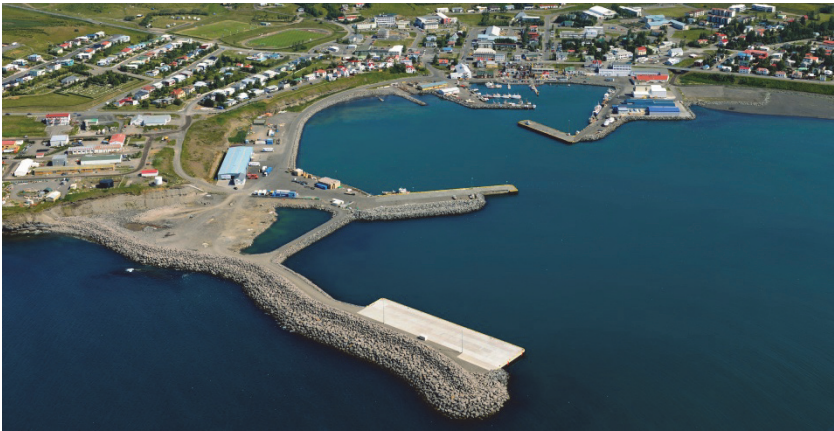
Figure 9.15. Husavik harbour in 2009. In the centre the 1988–1990 breakwater protects an older concrete pier. In the foreground the 2001–2002 breakwater. Photo by Mats Wibe Lund.
