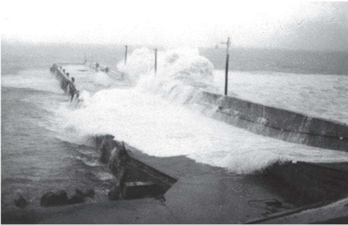
Figure 1.4. Overtopping during a storm at the pier of Hofsó before construction of the berm breakwater.
