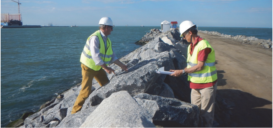
Figure 7.18. Measuring rock sides on the constructed armour layer.
