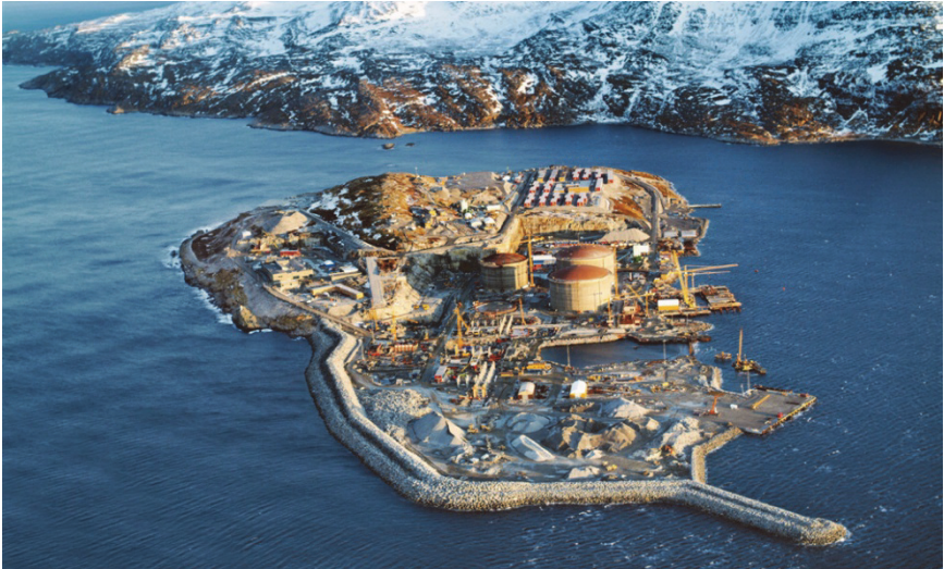
Figure 9.11. The Hammerfest LNG plant in November 2003. The breakwater revetment extends from the rocky shore in the centre left of the island to the breakwater head in the lower right hand corner and protects the plant area as well as the harbour. The most exposed part is leftward facing revetment. Courtesy of Statoil.
