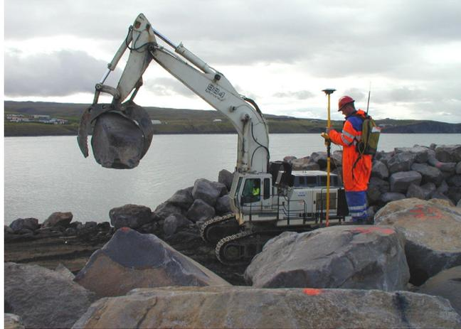
**Figure 1. From the construction of the Husavik berm breakwater. Surveying of class I armourstones, 16-30 tonnes, before building up the crest structure.**
