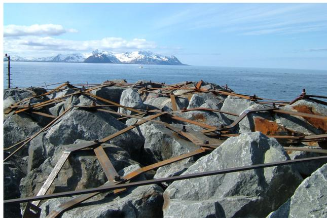
**Figure 2.** Temporary repairs after the 2002 storm included the bolting together of stones with steel bars.
