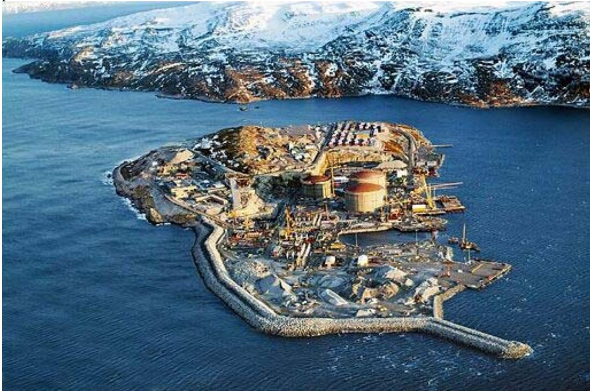
Figure 9. The Hammerfest LNG plant in November 2003 (courtesy of Statoil). The breakwater extends from the administration area in the centre left of the island to the breakwater head in the lower right hand corner and protects the plant area as well as the harbour. It is a combination of shore protection and freestanding breakwater.
