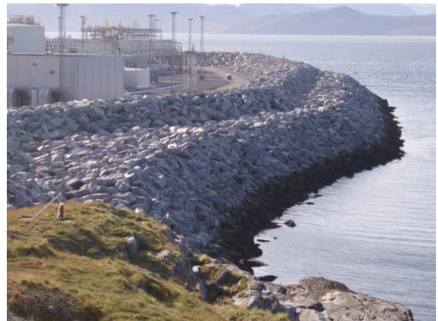
Figure 2 The Icelandic-type berm structure protecting the Hammerfest LNG plant, Norway. The porous high berm protects the rather vulnerable plant against overtopping and sea spray icing in arctic environment.
