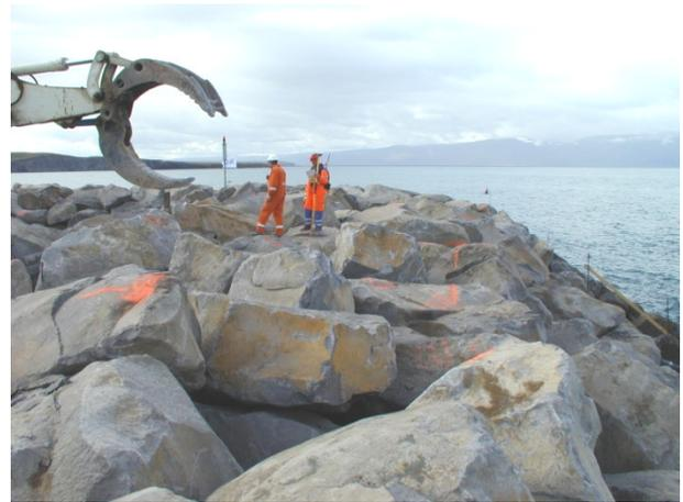
Figure 5 Surveying with a GPS staff of the Class I stones, 16 to 30 tonnes, of the berm at trunk and head sections before building the crest structure of the Husavik berm breakwater, Iceland.
