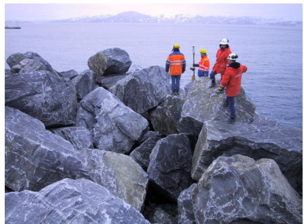
Figure 6 The Hammerfest breakwater, Norway, inspection survey with a GPS staff of the 20-35 tonnes Class I stone of the unfinished berm.
