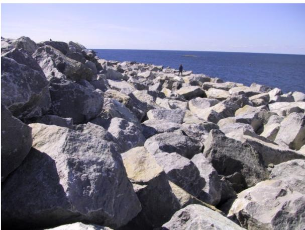
Figure 4 The Sirevåg berm breakwater, Norway, final inspection of the 20-30 tonnes Class I on berm.
