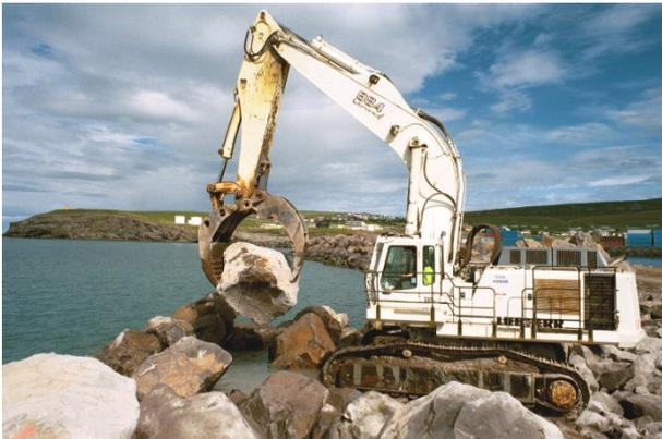
Figure 7 Excavator placing Class I 16-30 tonnes stones on the head of the Husavik berm breakwater, Iceland.
