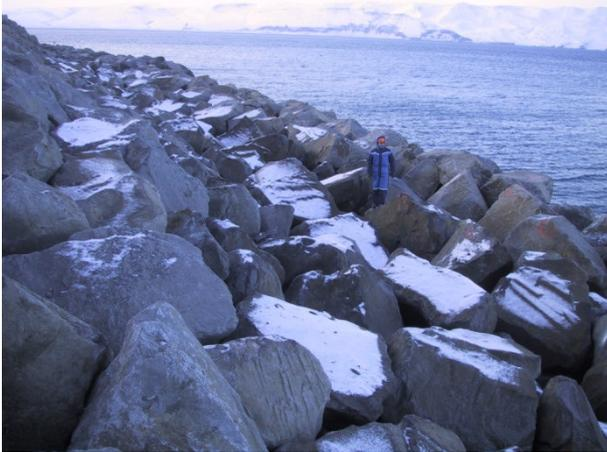
Figure 3 Narrowly graded stones on the Husavik berm breakwater, Iceland. Classes I and II, 16-30 and 10-16 tonnes. The photo clearly demonstrates the need to have a clear definition of the rock surface.
