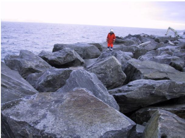
Figure 1 Class I stones, 20-35t on top of the Icelandic-type berm of the breakwater protecting the Hammerfest LNG plant, Norway.
