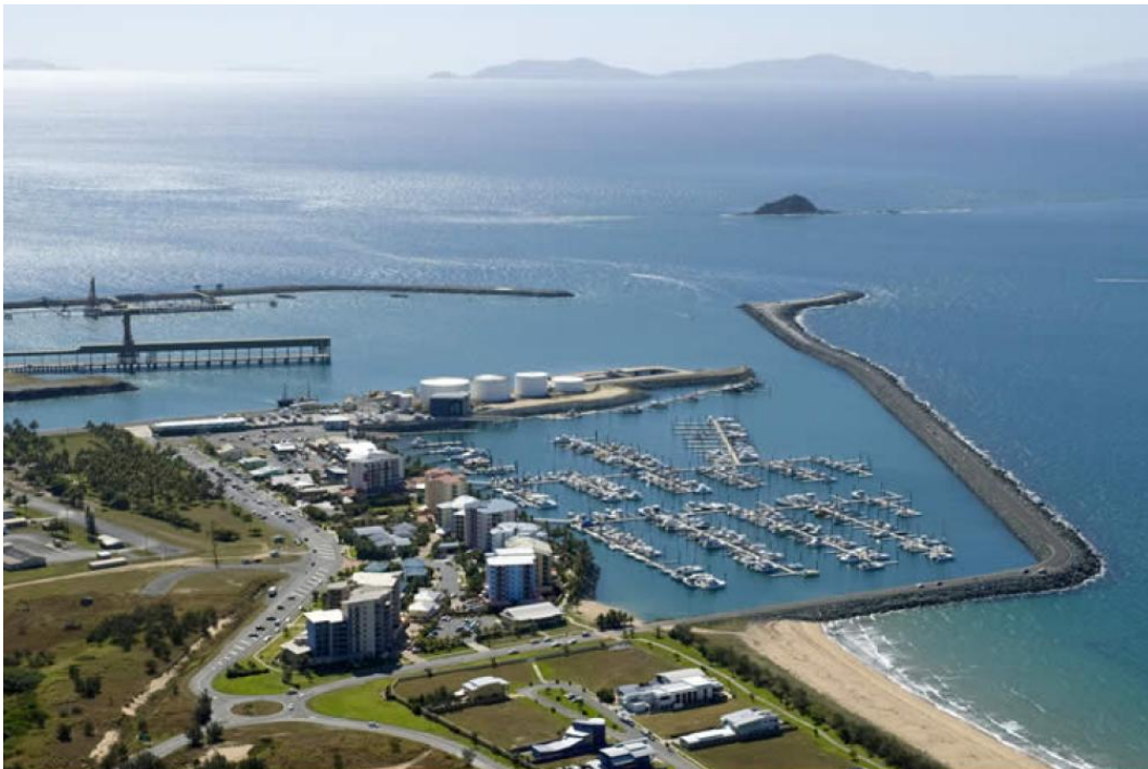
Figure 1. Mackay harbour, the Small Craft Harbour breakwater to the right on the photo protecting the marina, from NQBP (2011).
