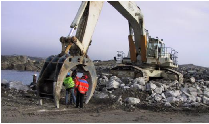
Figure 6. A 110 t excavator with a rock prong, Sirevåg breakwater.
