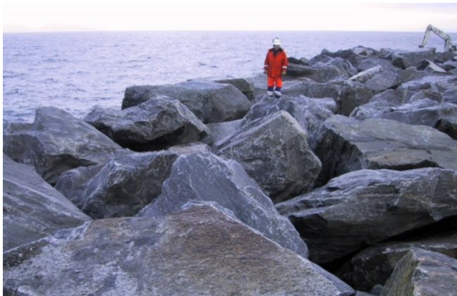
Figure 8. Class I stones, 20-35 t on the berm of the Hammerfest breakwater.
