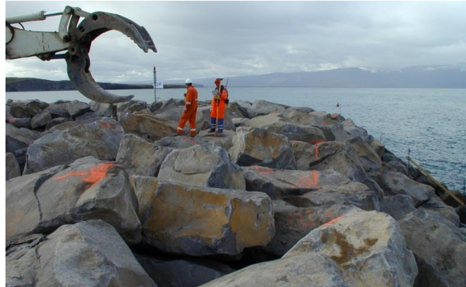
Figure 7: Surveying the Class I stones 16-30 t with a GPS staff on top of the berm of the Husavik berm breakwater, Iceland
