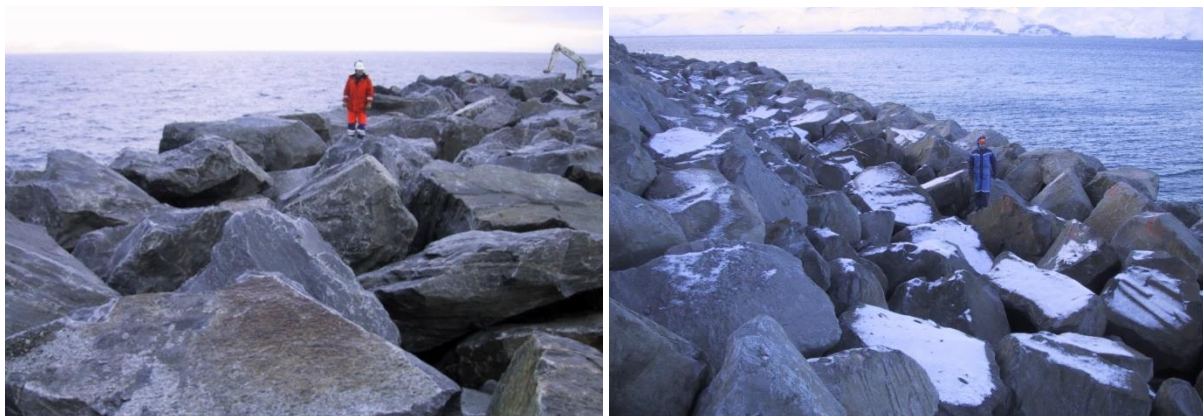
Figure 7: Class I stones, 20-35 t on the berm of the Hammerfest breakwater to left, and 16-30 t on the berm of the Husavik breakwater to right
