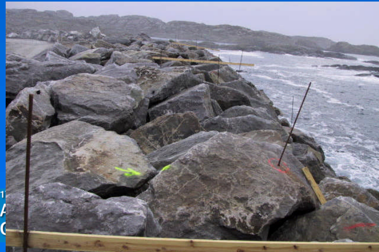
Figure 9.71 Effect of surveying methods on layer thickness for a double armour layer
